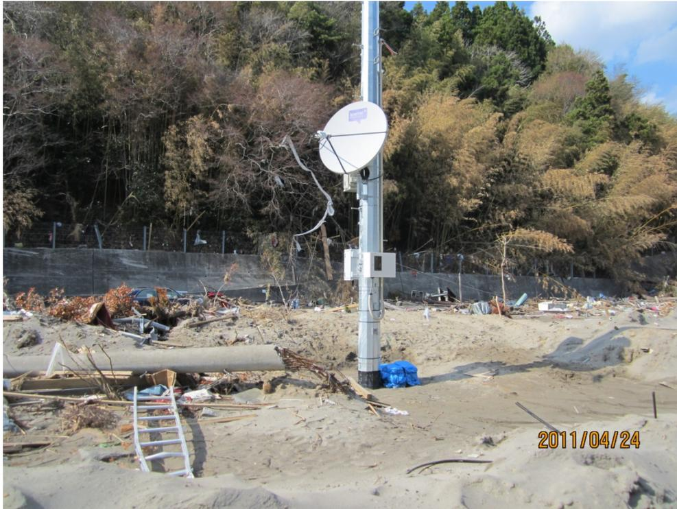
The persistent aftershocks foiled this otherwise excellent solution. For the accurate operation of the link from these remotely located cellular stations, a fixed satellite antenna requires the pointing accuracy to be maintained at all times. With each aftershock, many of the platforms would inevitably stop working due to pointing issues. The efforts of the Softbank team to provide cellular service to the people who so desperately needed it were, unfortunately, being wasted.
